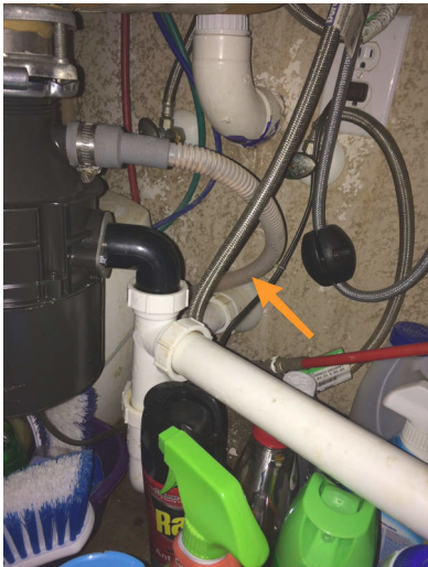
Dishwasher High Loop Drain Line
